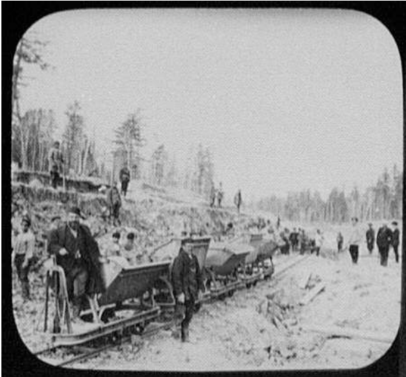
Construction Work on the Eastern Siberian Railway near Khabarovsk, 1895. http://hdl.loc.gov/loc.pnp/wtc.4a03376
